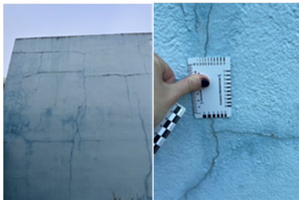
Fig. 4 Example of the current state of a Cité Frugès house’s polychromy and its analysis.
