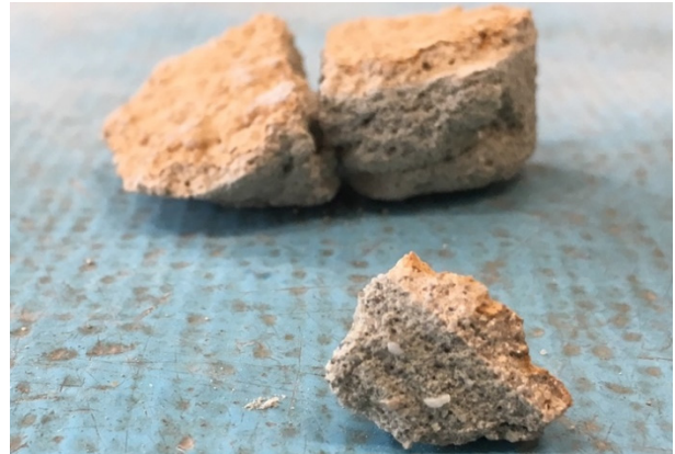
Fig. 3 Sample ASL_I taken from ex Asilo Santarelli building in Forlì.
