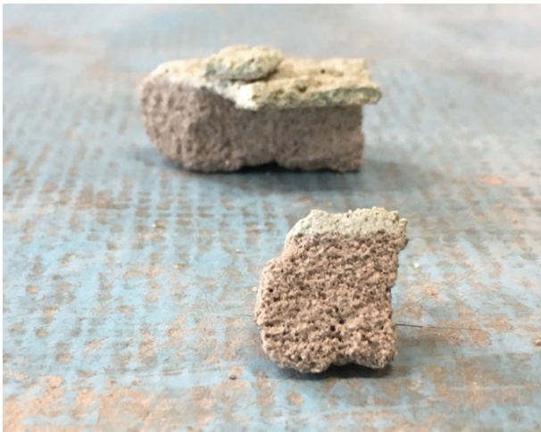
Fig. 1 Sample MOF_I taken from ex Mercato Ortofrutticolo (M.O.F.) building in Ferrara.
