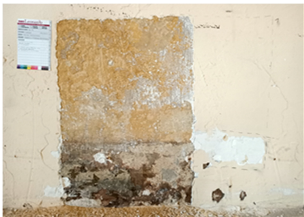
Fig. 7 Hall C, perimeter wall, sample No. 5: bichromy between the upper part, beige in color, and the brownish skirting ( Leonardo srl ).
